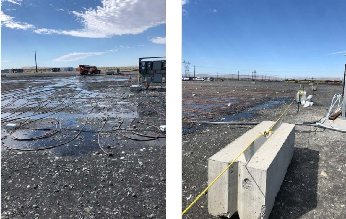
Figure 6. (left) Photograph taken during the first week of soil flushing in 2022, highlighting flush water distribution lines. (right) Photograph highlighting the ERT electrode array (white boxes connected by cables)
