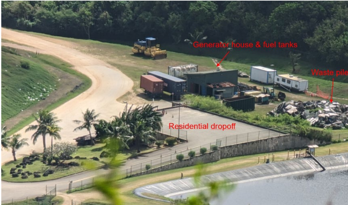
Figure 37. Overhead View of Potential Location Identified for Microgrid
