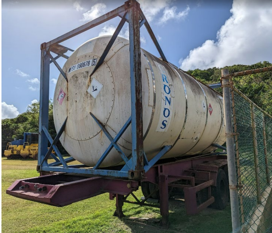
Figure 22. Portable Diesel Tank at Marpi Landfill
