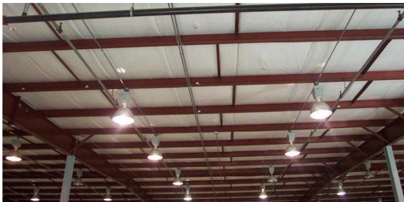
Figure 5012.4 Roof Insulation in Metal Buildings 2
