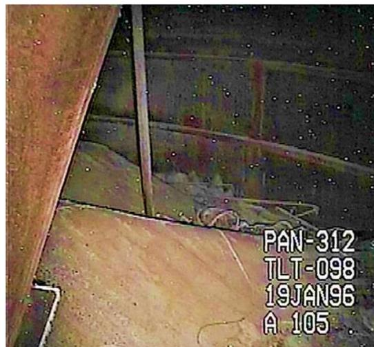
**Figure 3.2.** Liner Separated from Tank Wall
