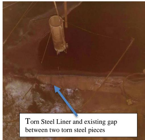
**Figure 3.1.** Tank A-105 Liner Bulge
