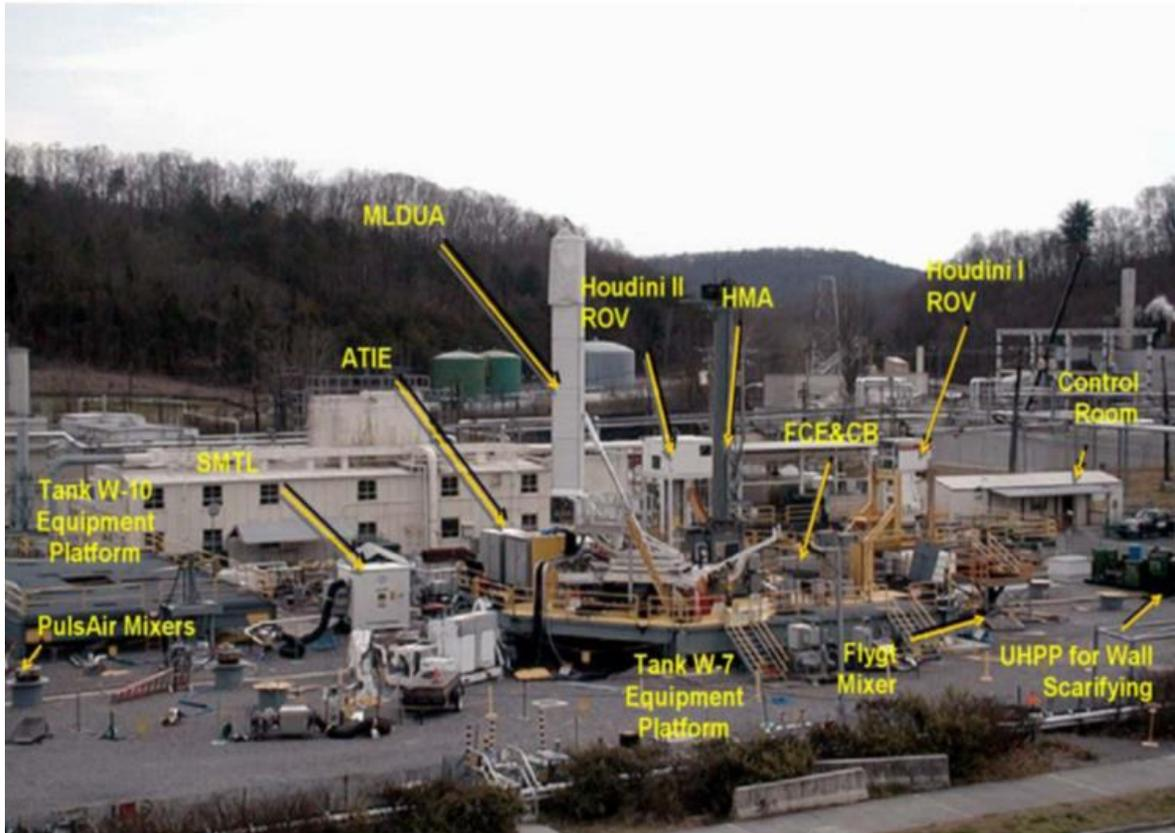
**Figure 2.2.** ORNL GAAT Retrieval Out-of-tank Support Systems including Deployment Systems
