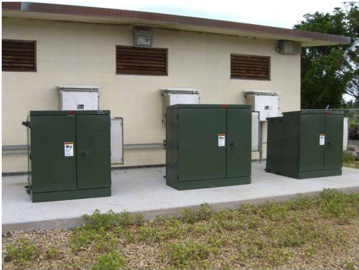
Figure 2.7. Outbound Modulation Units and Modulation Transfer Units at the MCBH Control Room
