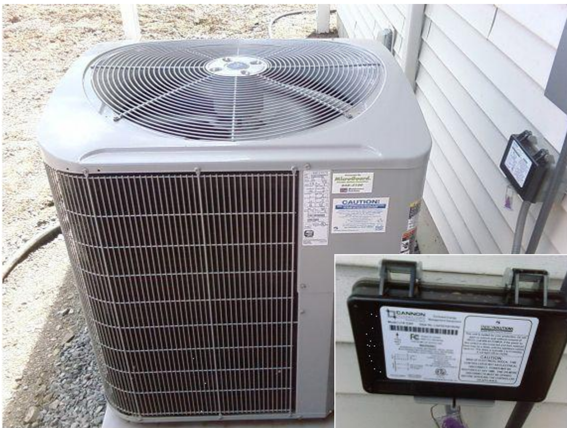
Figure 3.1. Air Conditioner with EnergyScout Canon Technologies Controller
