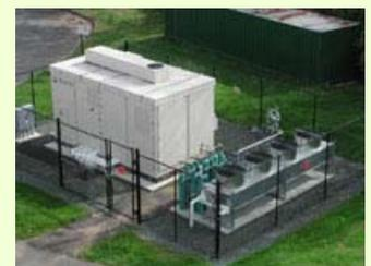
The fuel cell is interconnected to the school's electrical, heating boiler, make-up air, and potable water systems. Before the installation of the fuel cell, natural gas was not available on site. Consequently, natural gas service had to be added as part of the installation.
